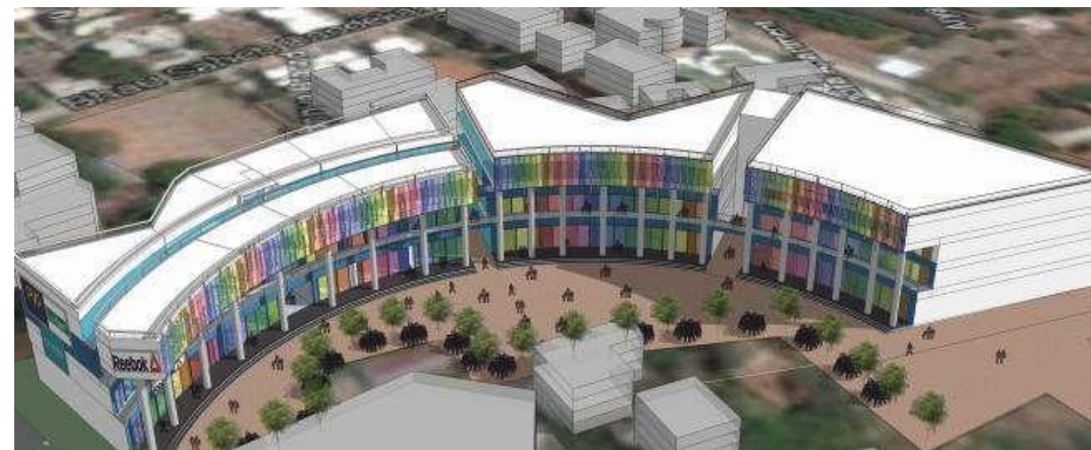
Commercial development at Palghar Maharashtra
